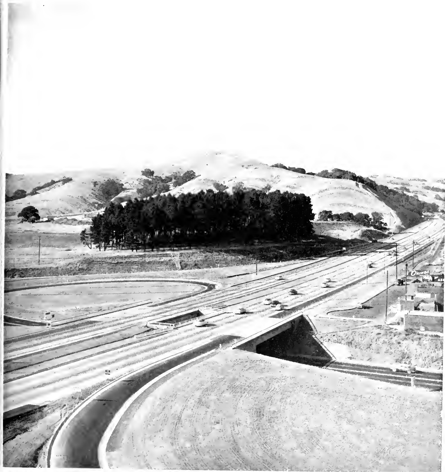
This is the new Orindo Interchange on Sign Route 24 in Contra Costa County
